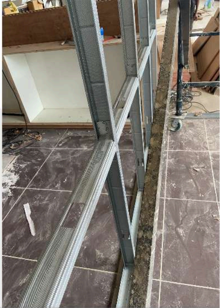
Server Room, Baner Pune (2 hr Fire Partition Wall)
