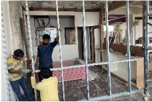
Server Room, Baner Pune (2 hr Fire Partition Wall)
